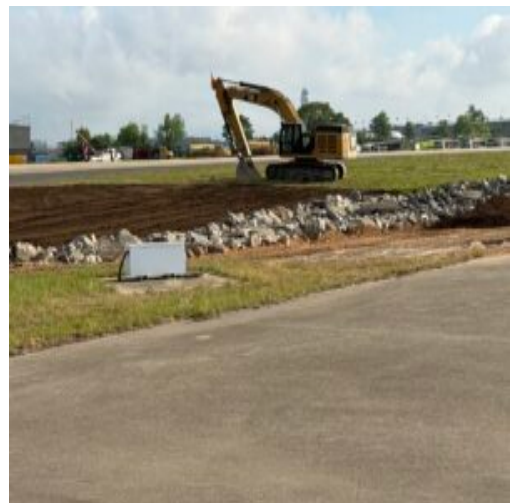
spreading topsoil
