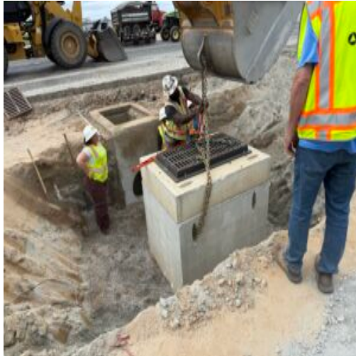
Area 1 box placement
