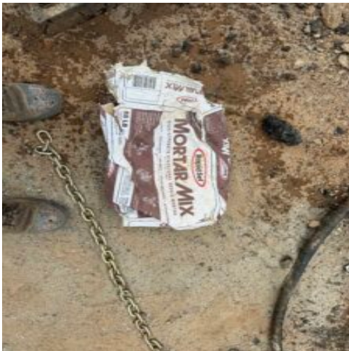
Mix used to for collar area 1 drain
