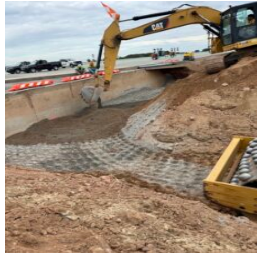
Backfilling Area 4
