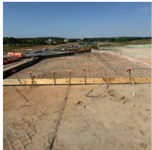
New concrete area
