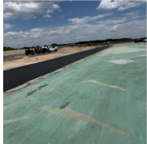
Asphalt paving Area 1
