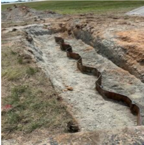
Sheet piles cut below grade
