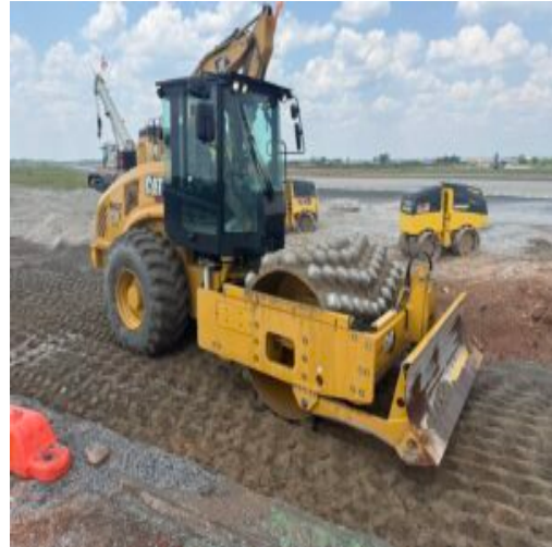
compacting final lift
