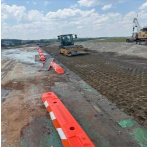
compacting final lift
