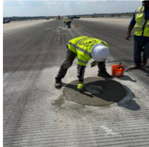
Placing concrete around light cans center runway.
