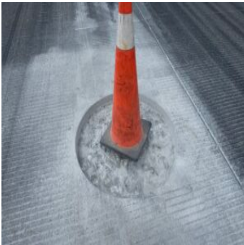
light cans cored before concrete placement
