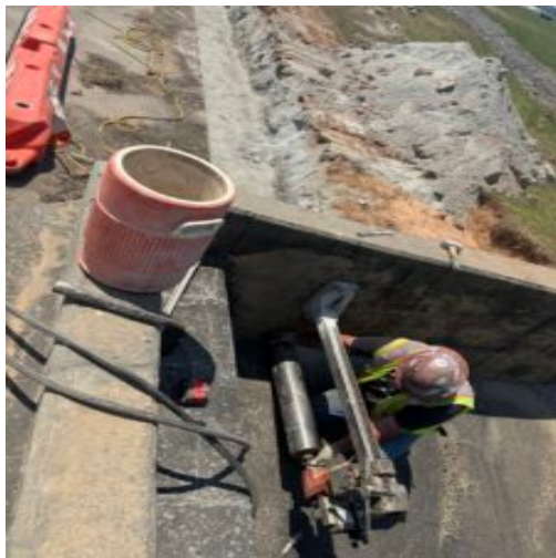
Area 5 Hole drilled through wall for drain
