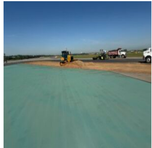
Preparing for GAB Area 1
