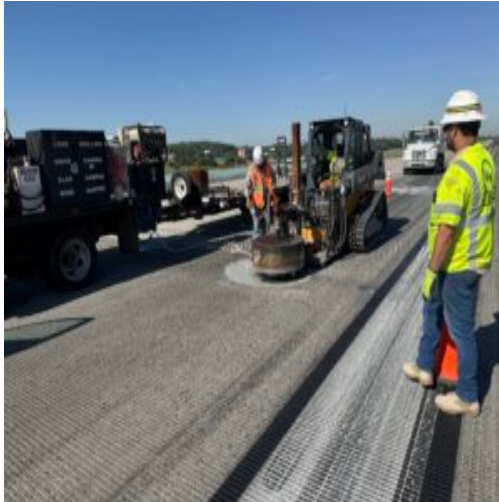
Coring around existing Lights
