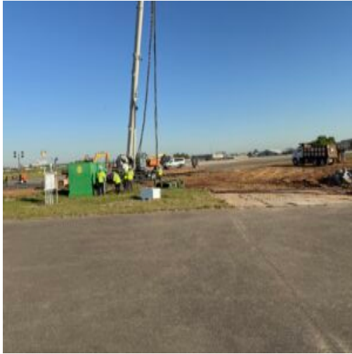
Sheet pile installation
