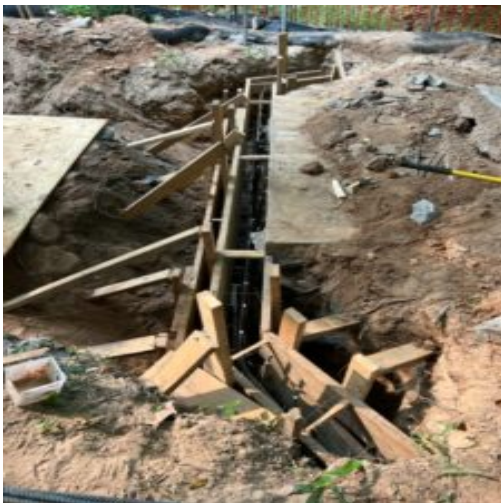
Rebar and formwork before placement
