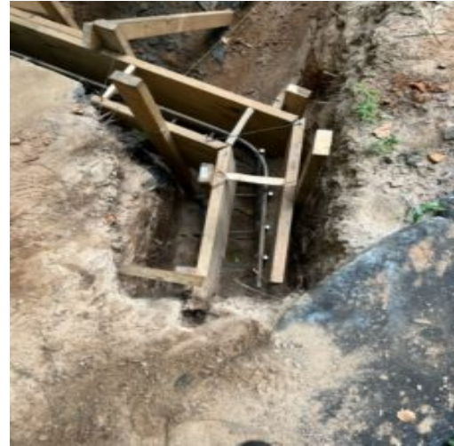
Rebar and formwork before placement
