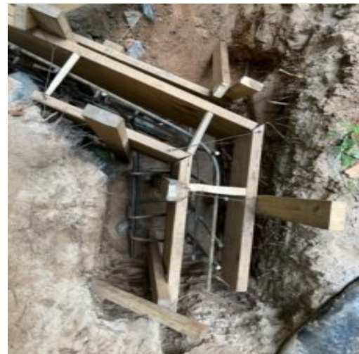
Rebar and formwork before placement
