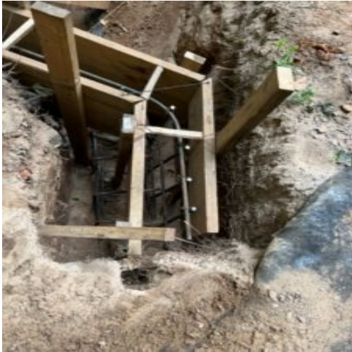
Rebar and formwork before placement
