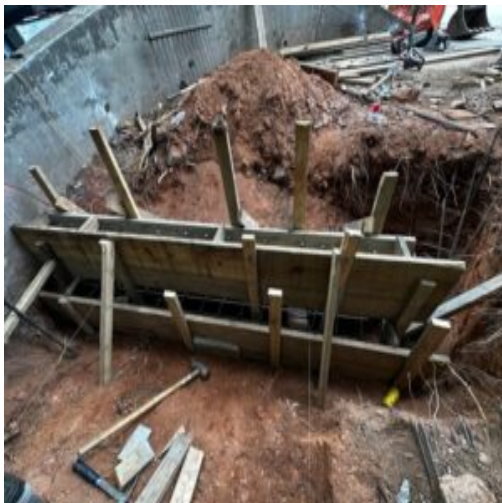
Rebar and Formwork at the placement
