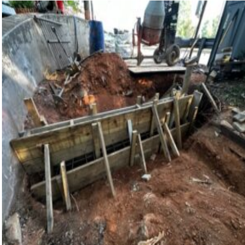
Rebar and Formwork at the placement
