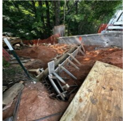
Rebar and Formwork at the placement
