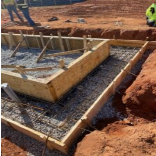
Rebar and Forms for Vault 2 foundations
