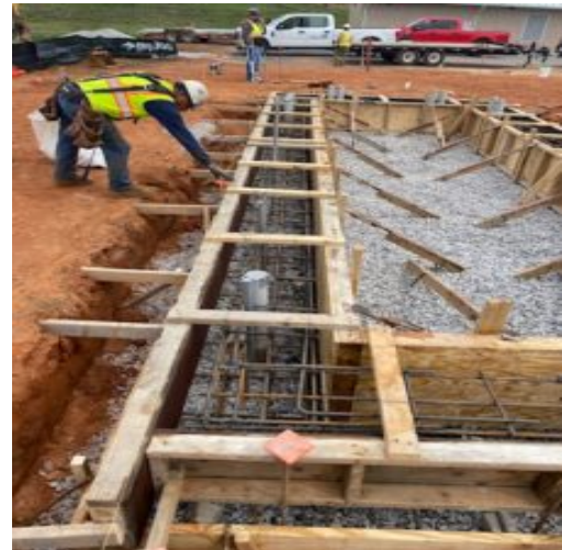
Rebar and Forms for Vault 2 foundations
