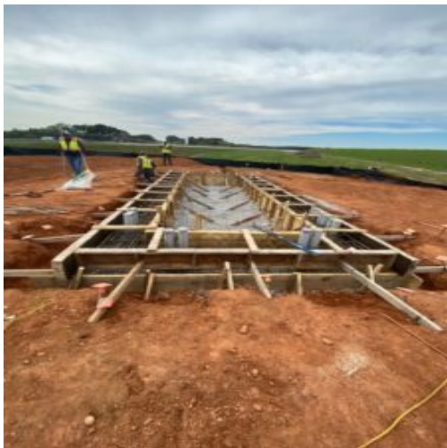
Rebar and Forms for Vault 2 foundations
