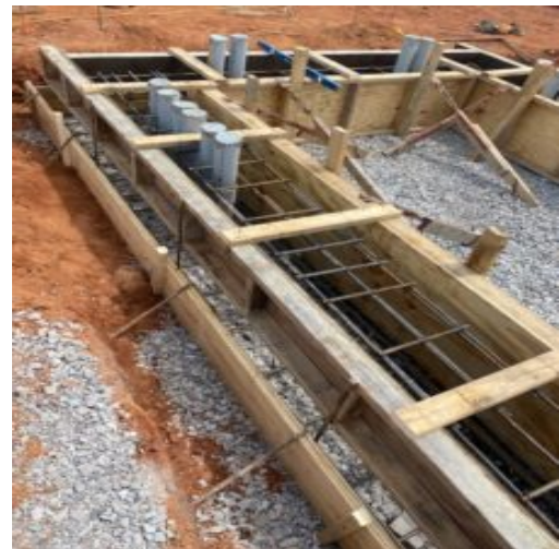
Rebar and Forms for Vault 2 foundations
