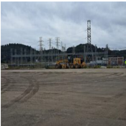
Leveling of 825-B stone on the basement
