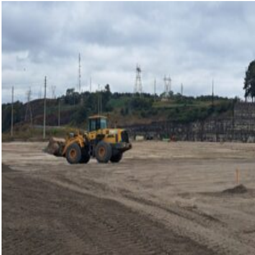
Leveling of 825-B stone on the basement
