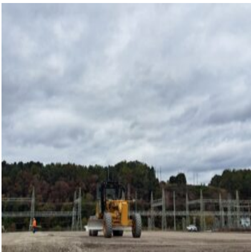
Leveling of stone
