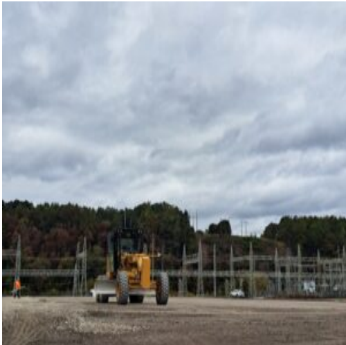
Leveling of stone
