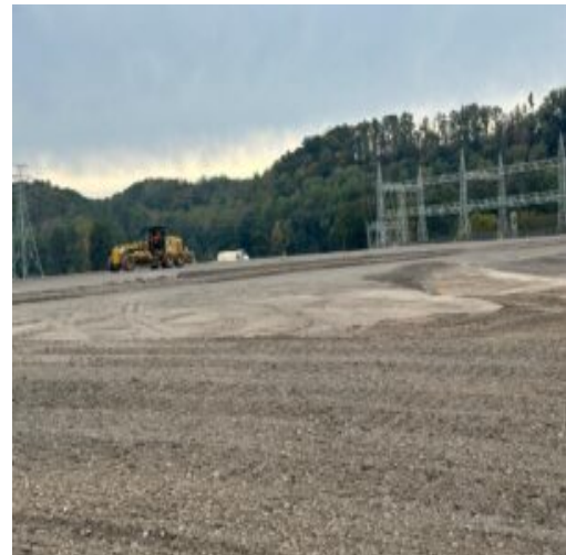
Spreading of 825-B stone
