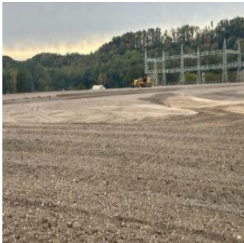
Spreading of 825-B stone
