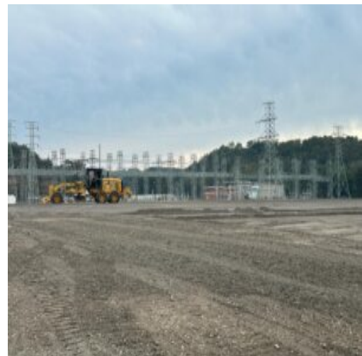
Compaction of 825B material being performed
