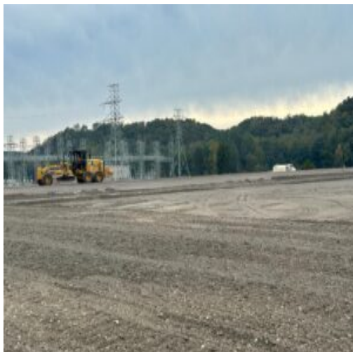
Compaction of 825B material being performed
