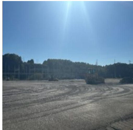
Spreading of 825-B stone
