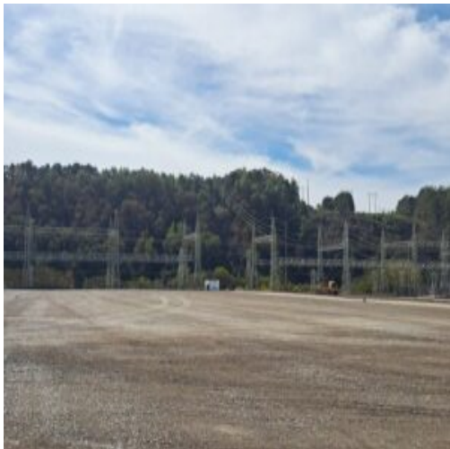
Placed the 825-B Stone in basement
