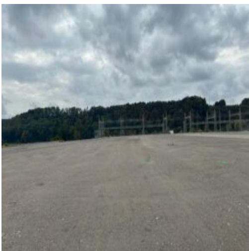
Basement is placed with 825-B stone in basement
