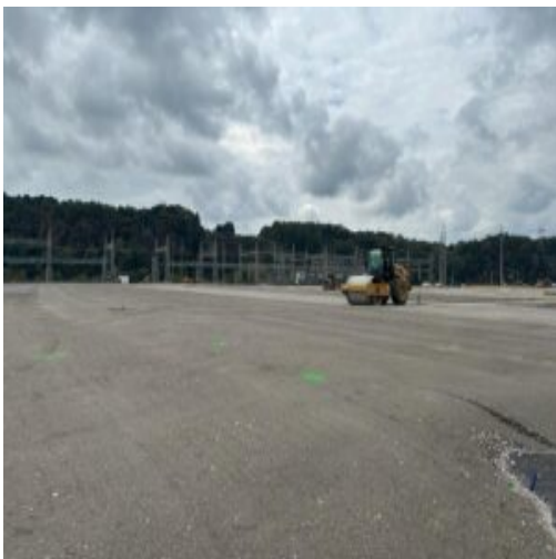
Compaction of 825B material being performed
