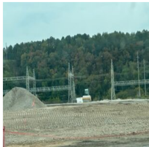
Dozing is performed on the basement
