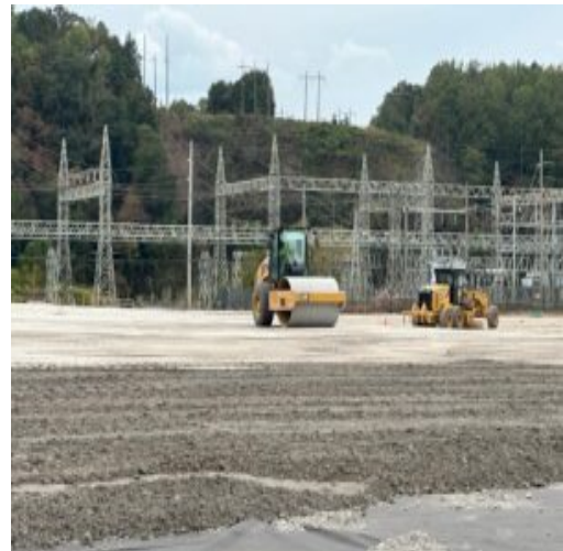
Dozing is performed on 825-B stone
