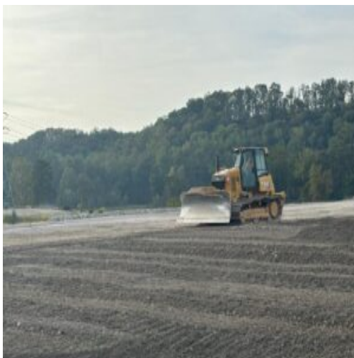
Hauling is performed on the basement
