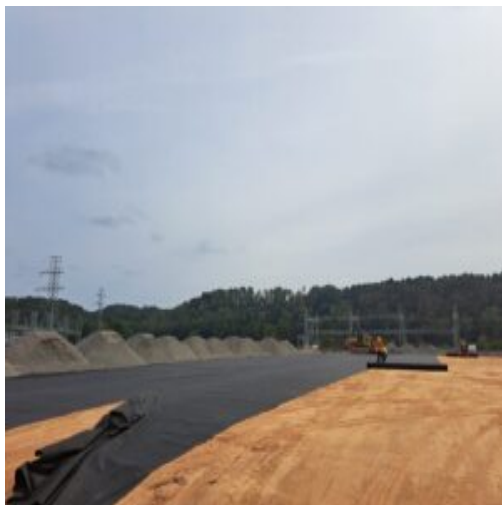
Geo-fabric is placed on other side of basement
