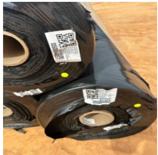
Geo-fabric has been received
