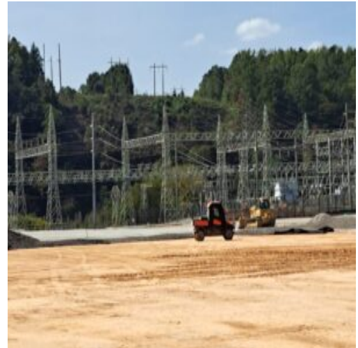
Dozing is performed on the 825-B stone
