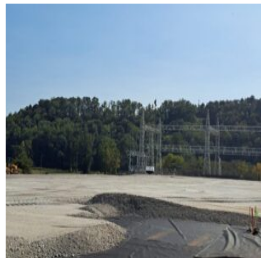
Placing of stone material in basement
