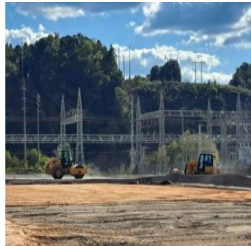
Dozer is performed in the basement
