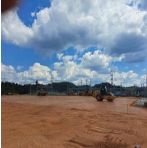
Leveled the soil using the roller
