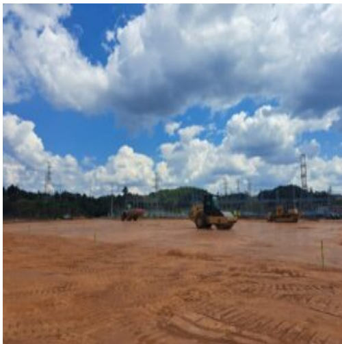
Leveled the soil using the roller
