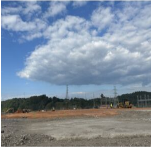
Placed the soil in the basement
