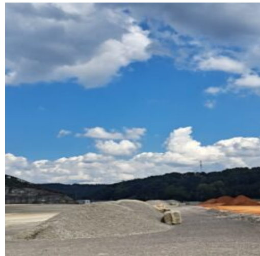
Received the crushed concrete to the site
