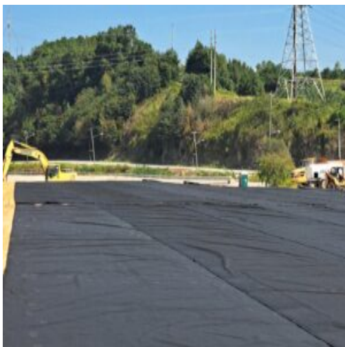
Spread the geo-fabric on the site
