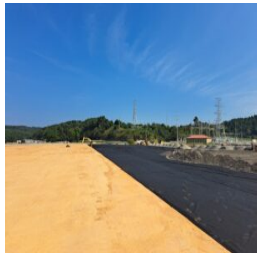
Placed the 825-B Stone above the fabric
