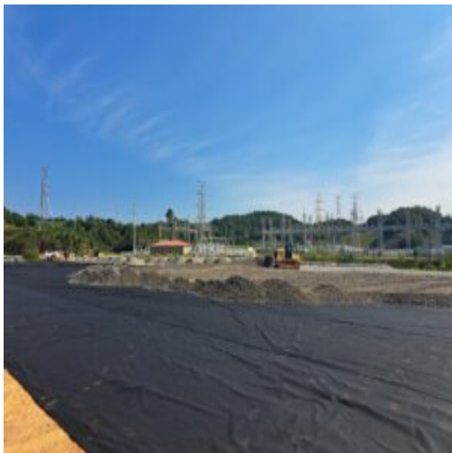
Placed the 825-B Stone above the fabric
