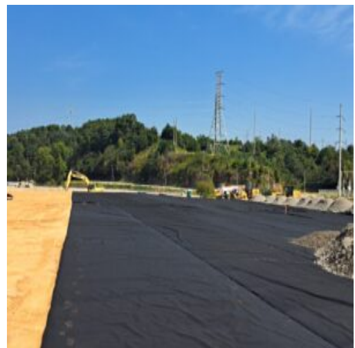
Placed the 825-B Stone above the fabric
