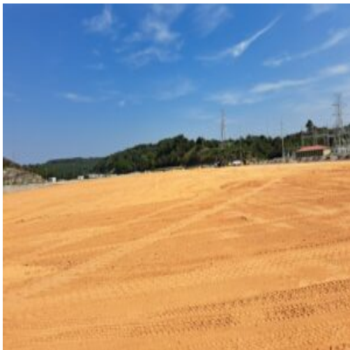
Hauling in the basement area
