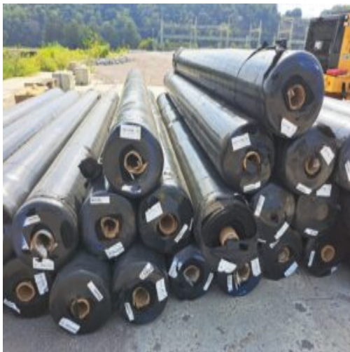
Geo-fabric received on site
