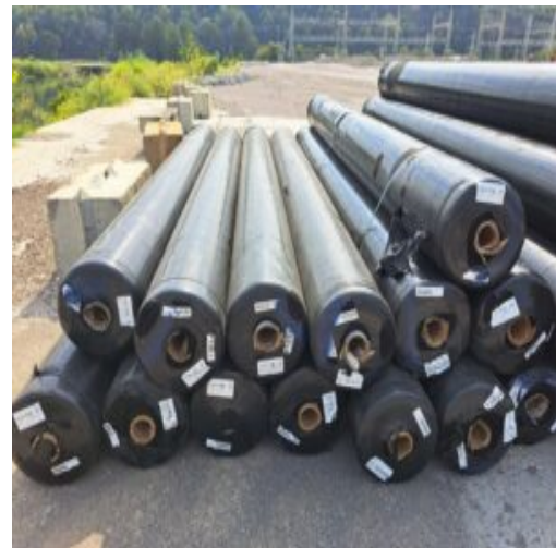
Geo-fabric received on site
