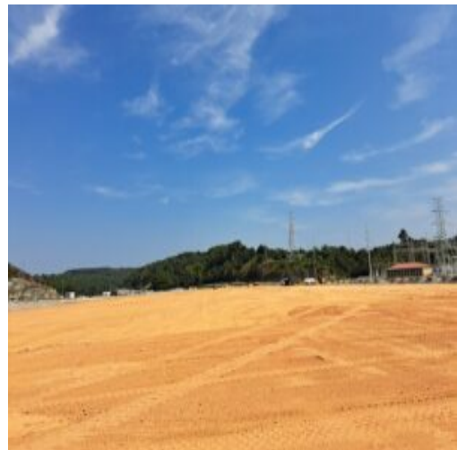
Hauling in the basement area
