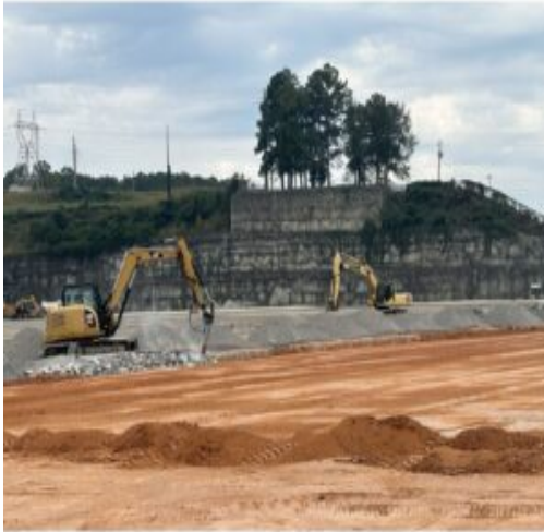
Crushing of stones in section 1
