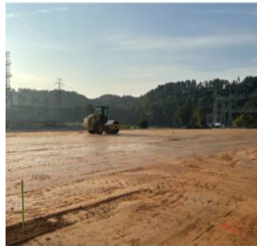
Leveling the fill material using the Dozer
