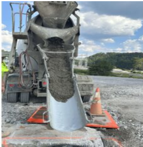
Poring the flowable fill in the HDPE pipe
