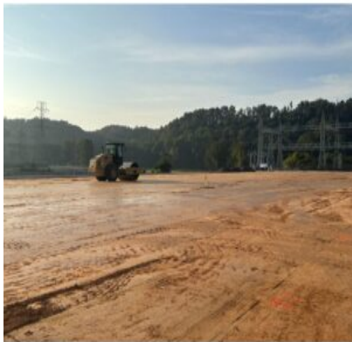
Leveling the fill material using the Dozer
