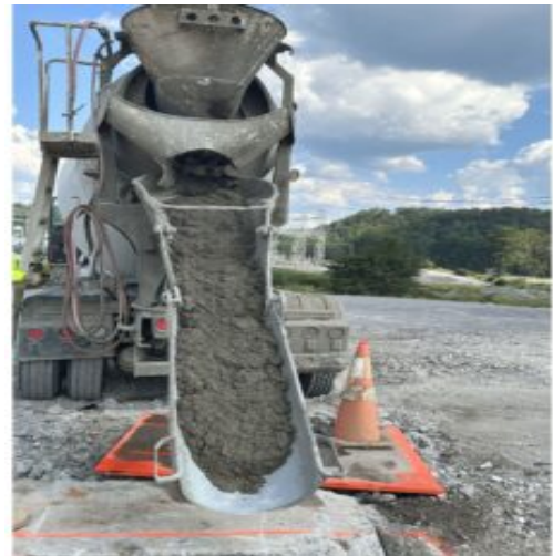
Poring the flowable fill in the HDPE pipe
