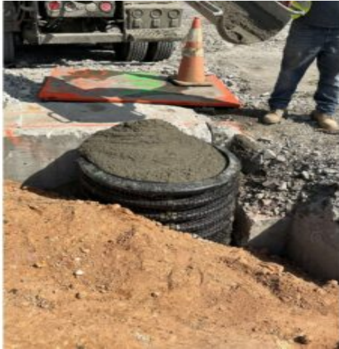
Completely filled HDPE pipe with Flow-fill
