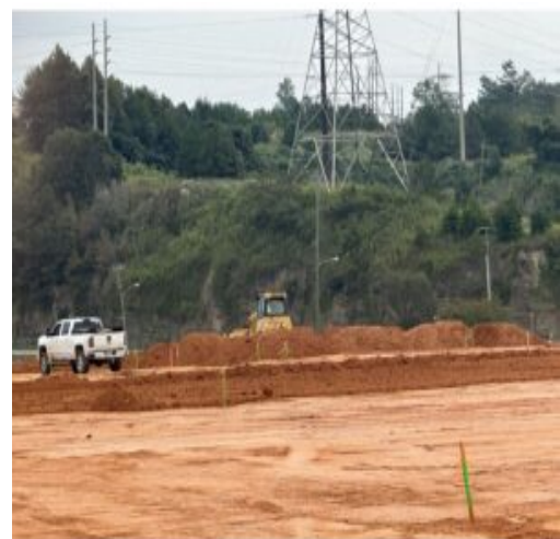
Fill materials were placed in section 1
