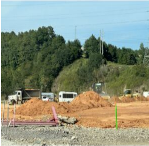
Structural fill materials placed on section 2
