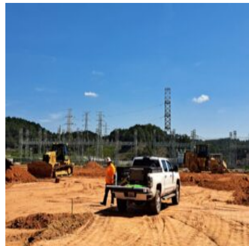
Lift is placed on section 2
