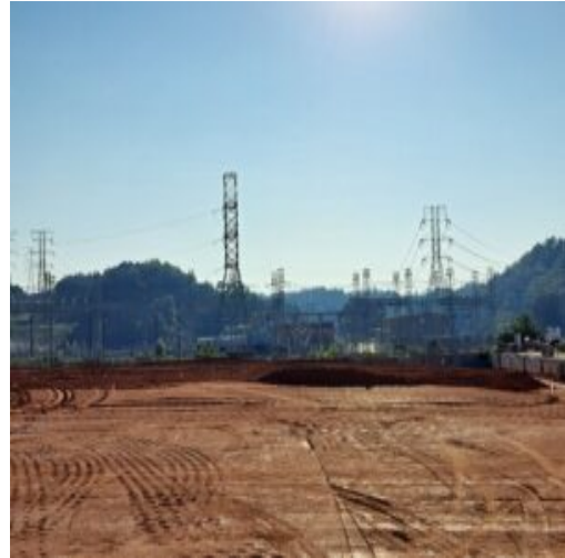
placed the structural fill materials in Section 2
