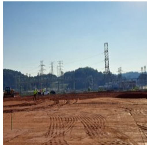
Placement of structural fill materials in section 2
