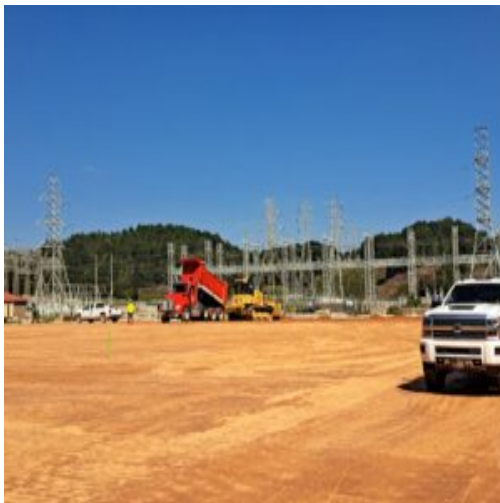
Placement of structural fill material in section 2
