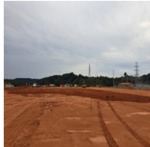
Placement of structural fill material in the section 2 part 2 Placed the structural fill materials in section 1 and section 2 part 1
