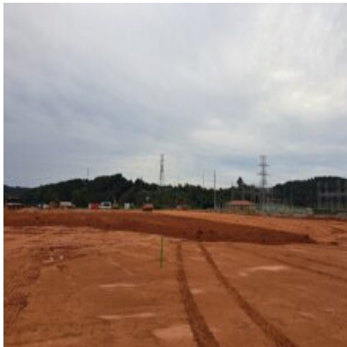
Placed the structural fill materials in section 1 and section 2 part 1 Placed the structural fill materials in section 1 and section 2 part 1
