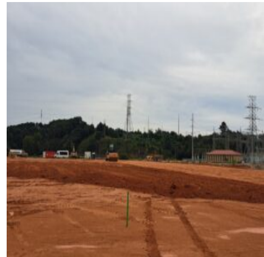
Placed the structural fill materials in section 1 and section 2 part 1 Placed the structural fill materials in section 1 and section 2 part 1
