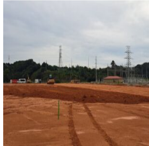
Placed the structural fill material in section 1
