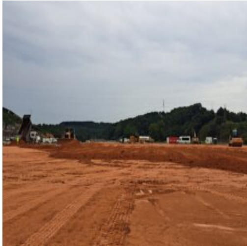
Placed the structural fill material in section 1
