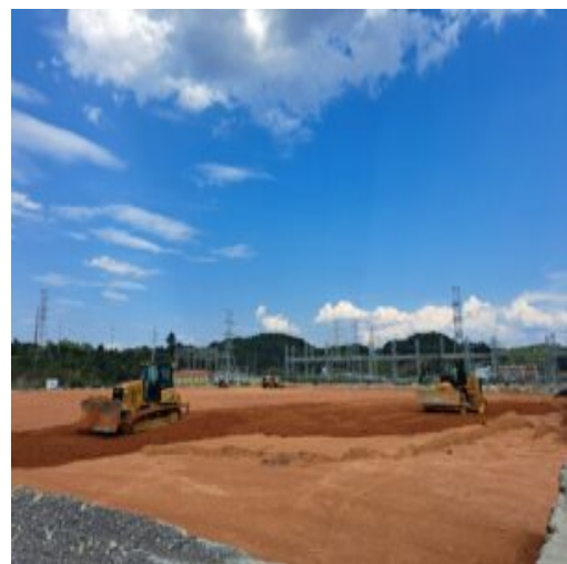
Lift is placed on section 1
