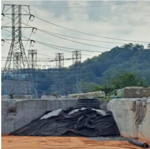
Covered HDPE pipe with Geo-fabric
