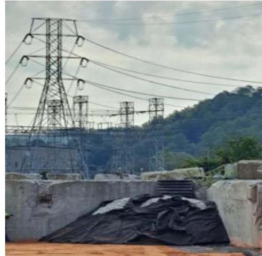
Covered HDPE pipe with Geo-fabric
