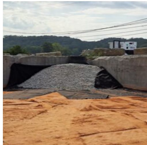
Placed the stone-aggregate around the pipe
