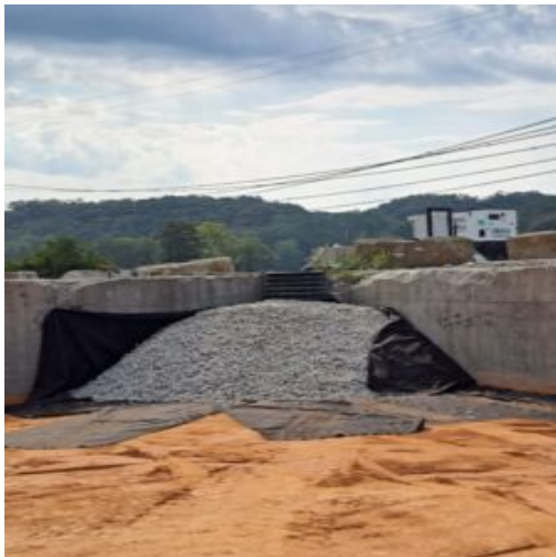
Placed the stone-aggregate around the pipe
