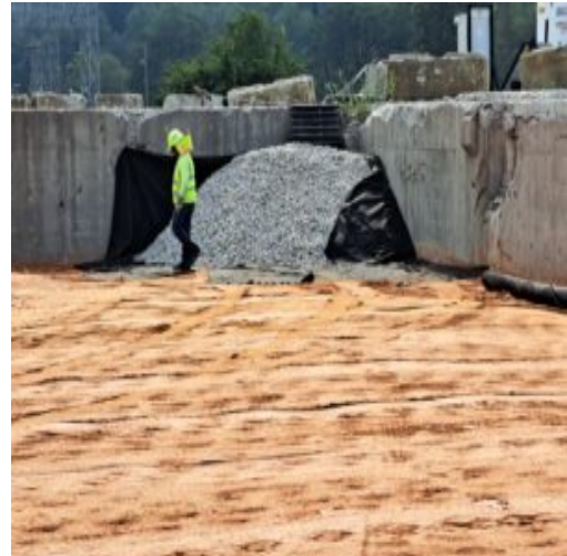
Placed the stone-aggregate around the pipe
