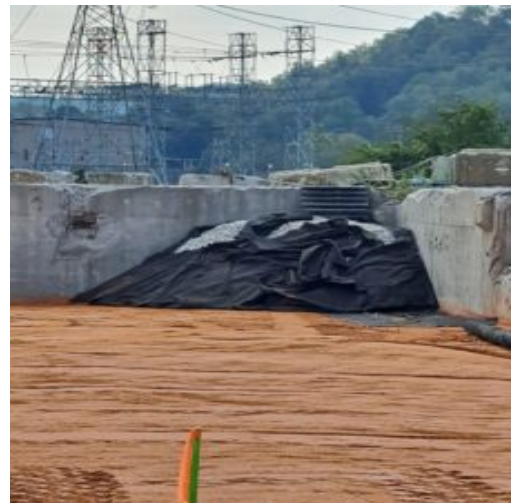
Covered HDPE pipe with Geo-fabric
