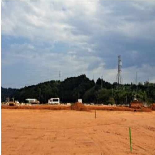
Placement of structural fill material in section 1
