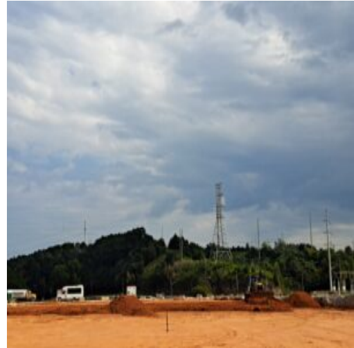
Placement of structural fill material in section 1
