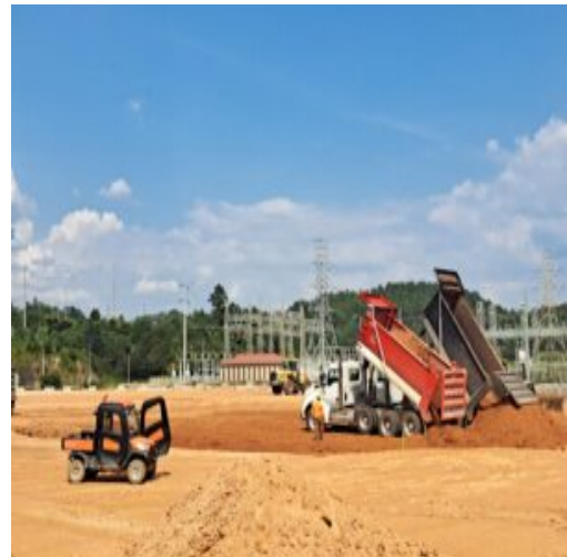
Placement of structural fill material in section 2 basement area
