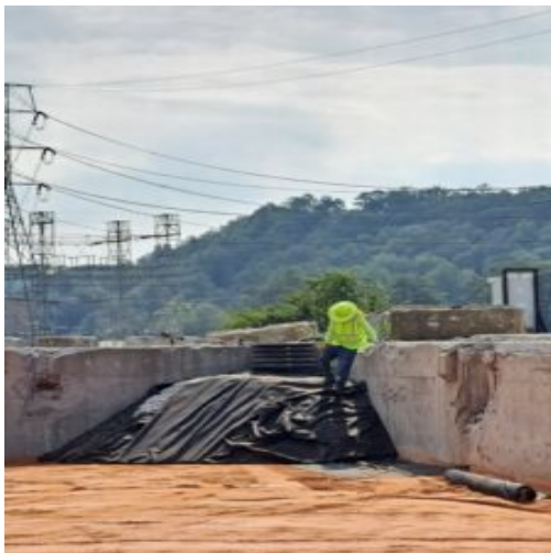
Covered HDPE pipe with Geo-fabric
