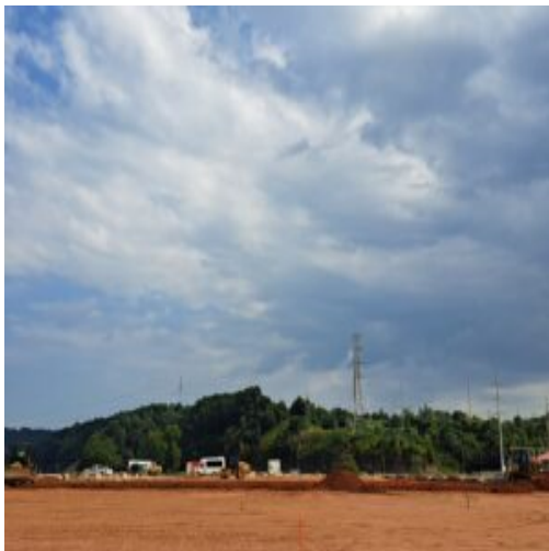
Placement of structural fill material in section 1
