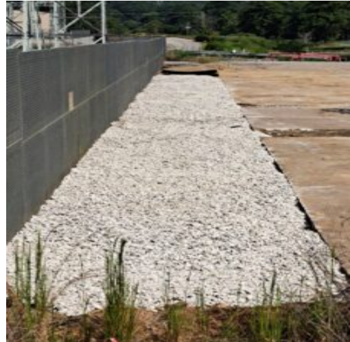
Rock Boulders has been placed on the topmost of all the materials
