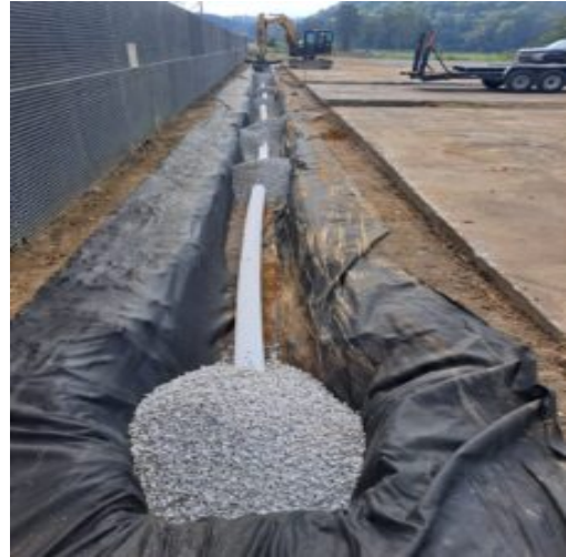
Pipe has been installed in french drain water treatment area
