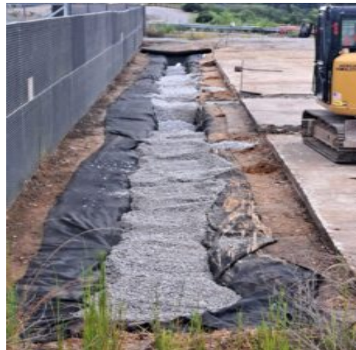
Stone aggregate has been placed on the top of the pipe
