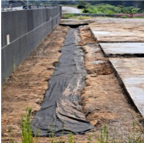
Geo-fabric has been installed to cover the stone aggregate
