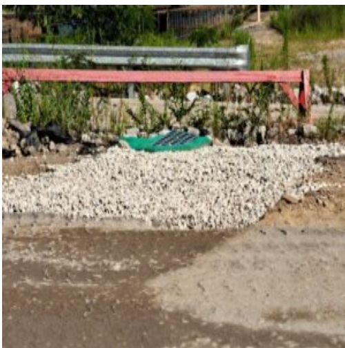
Placed 57-Stone along the trench drain water treatment area
