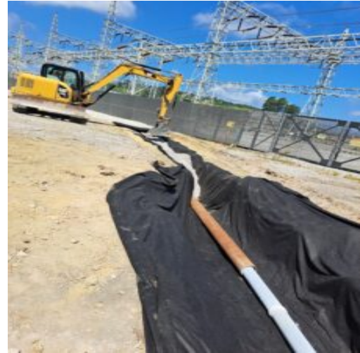
Placed aggregate in the trench after the placement of HDPE pipe was placed in the trench after the Geo-fabric placement.
