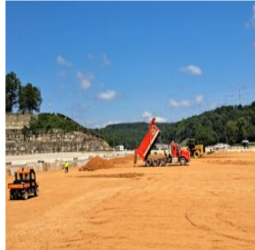
placement of structural fill materials in section near the ramp
