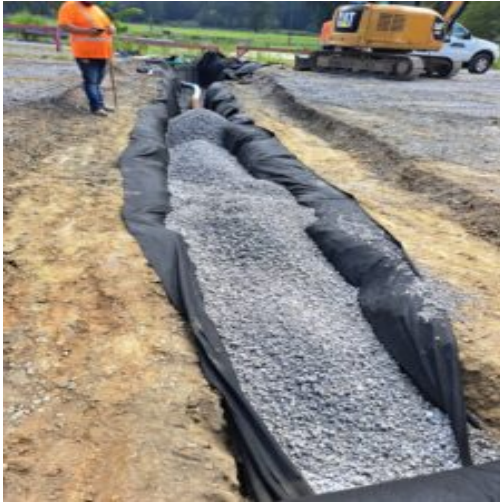
Placed aggregate in the trench after the placement of HDPE pipe was placed in the trench after the Geo-fabric placement.
