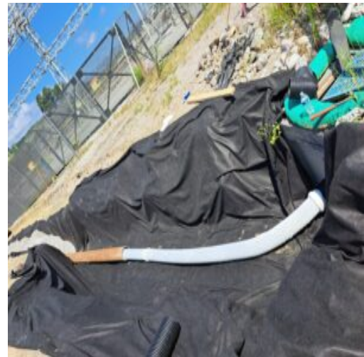
HDPE pipe was placed in the trench after the Geo-fabric placement.
