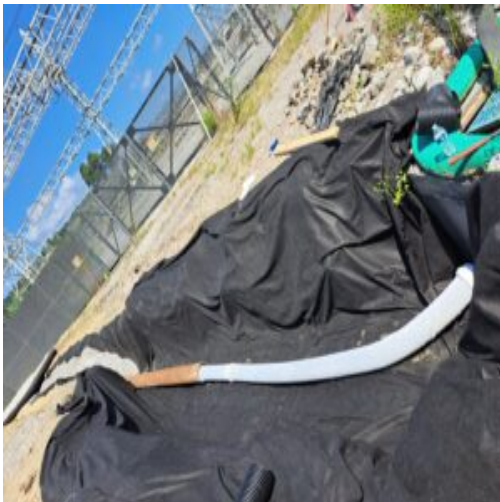
Perforated pipe was placed in the trench after the Geo-fabric placement.
