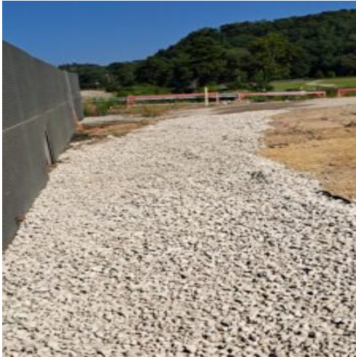
Placed 57-Stone along the trench drain water treatment area
