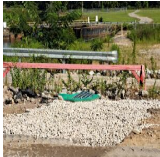
Placed 57-Stone at trench drain water treatment area
