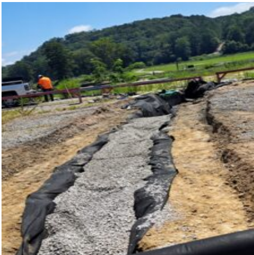
Placed aggregate in the trench after the placement of perforated pipe
