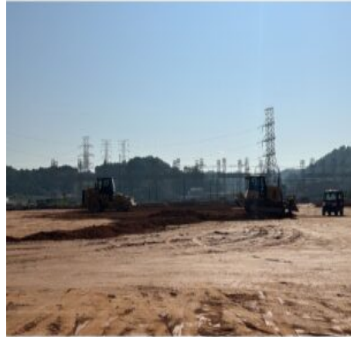
Lift is placed on section 2 part 1
