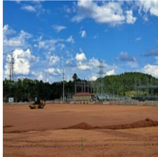
Hauling of structural field material in section 2
