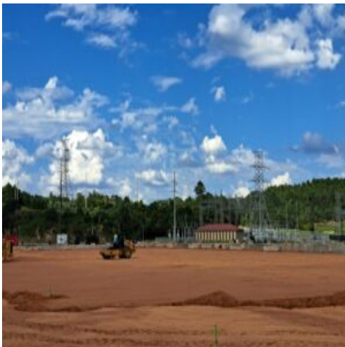
Lift is placed on section 2
