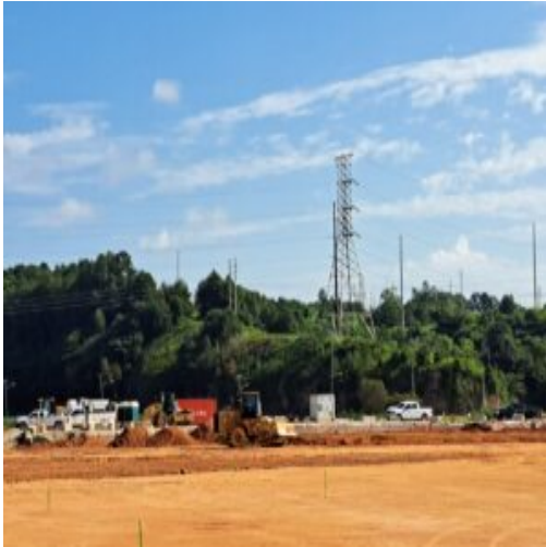
Lift is placed on section 1
