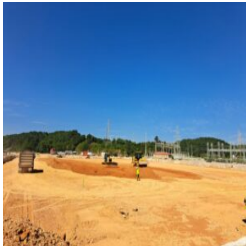
Lift is placed in section 2
