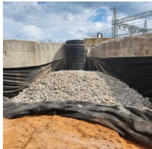
Placed the stone before the coverage of Geo-fabric
