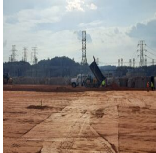
Placement of fill-material in section 2
