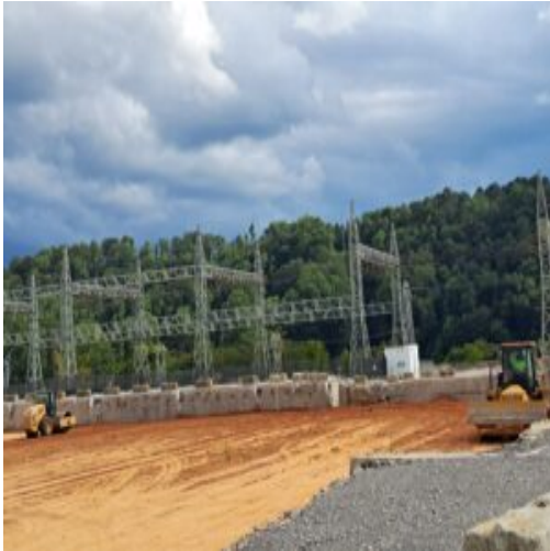
Placement of fill-material in section 2
