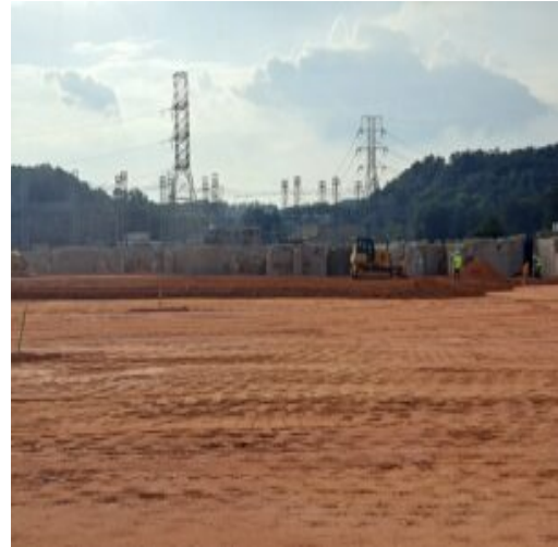
Placement of fill-material in section 2
