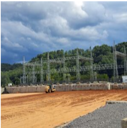
Placement of fill-material in section 2
