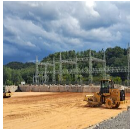
Placement of fill-material in section 2
