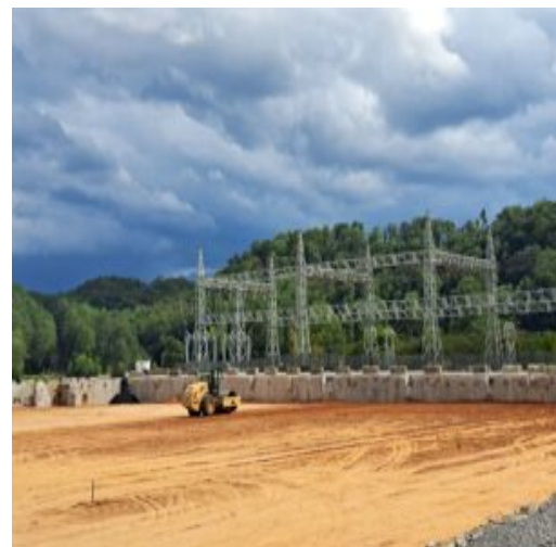
Hauling and compacting in section 2
