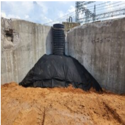
Covered the HDPE with Geo-fabric
