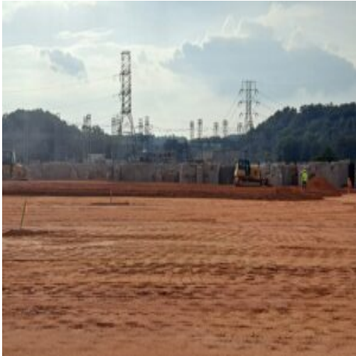
Placement of fill-material in section 2
