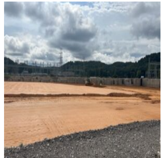
Lift being placed and compacted
