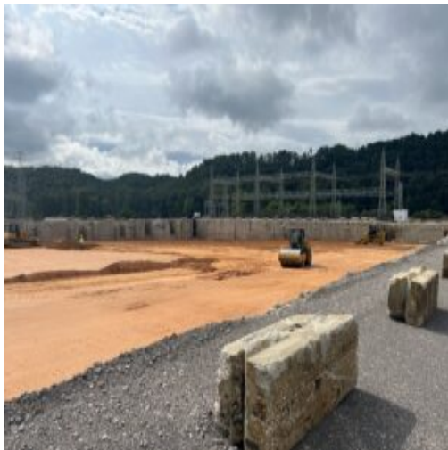
Smooth drum roller to seal off the placed common fill
