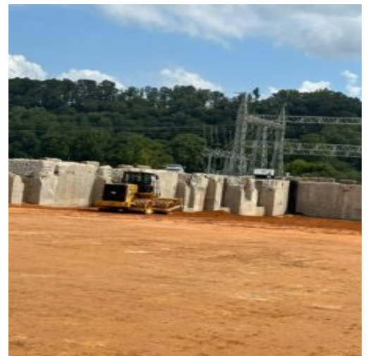
Continued compacting fill using an 815
