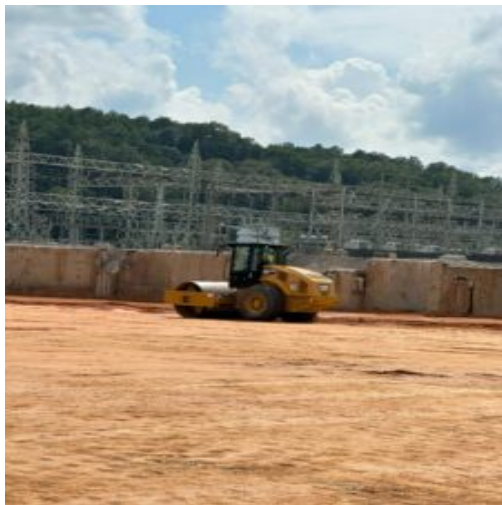
Smooth drum roller sealing areas that have been compacted using a 815.
