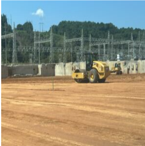
Spreading material in approximately 12 inch loose lifts
