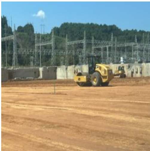
Smooth drum roller performing sealing operation due to impending rain.
