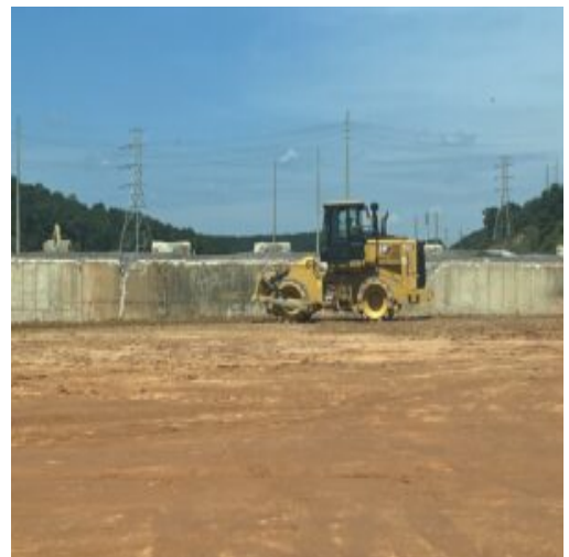
Compaction efforts using an 815 compactor
