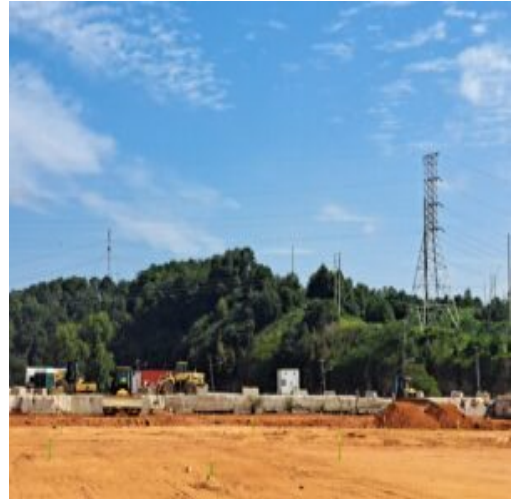
Lift is placed in section 1
