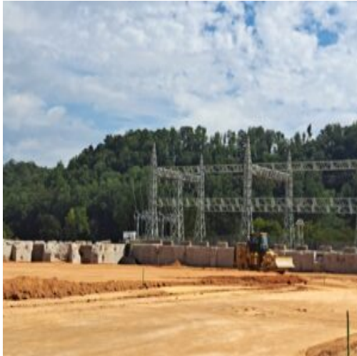
Lift is placed in section 2 part 1
