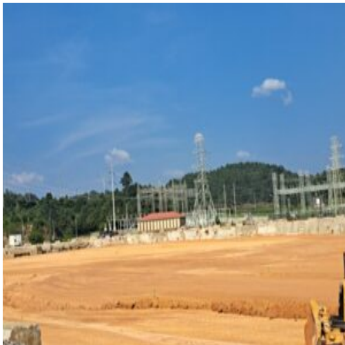
Lift is placed on section 2 part 1
