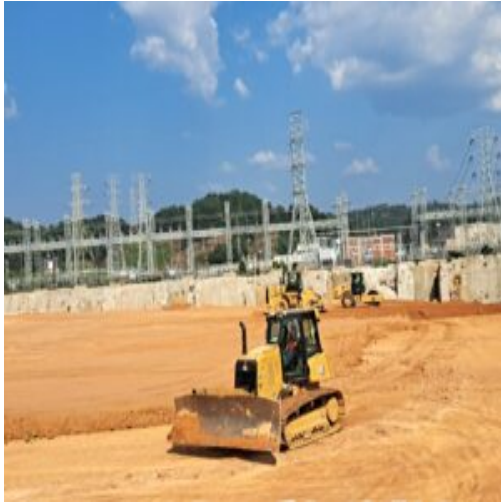
Hauling is performed on fill material in section 2 part 1
