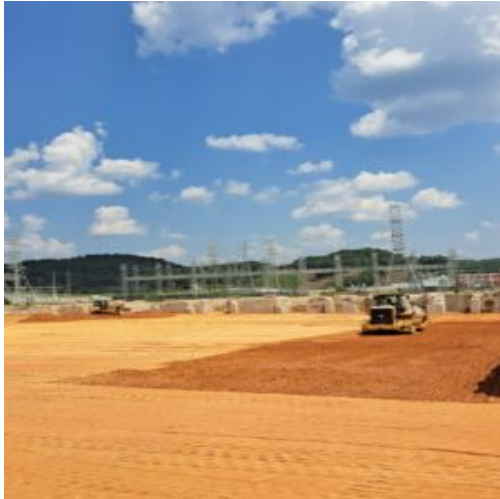
Hauling the fill materials in section 2
