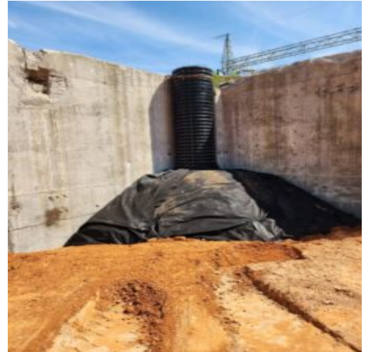
Covered HDPE with Geo-fabric
