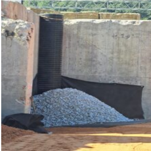
Placed Geo-fabric around HDPE Pipe
