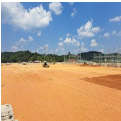
Placement of fill materials in section 2
