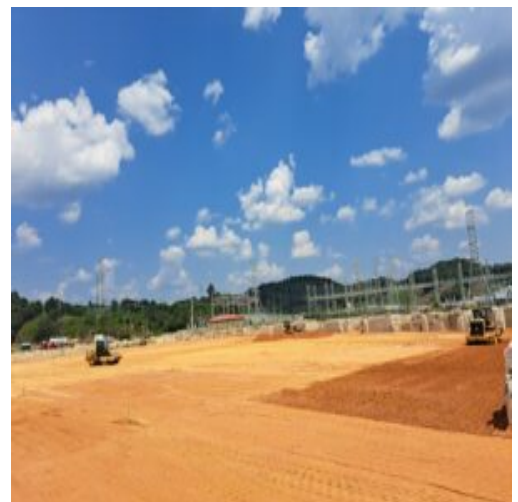
Placement of fill materials in section 2
