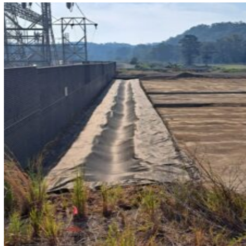
Geo fabric is placed in French Drain Water treatment area
