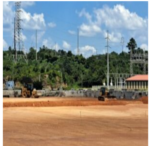
Placement of Lift at section 2 part 2
