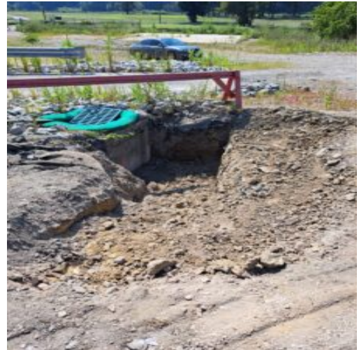
Trench has been excavated at the depth of 2ft
