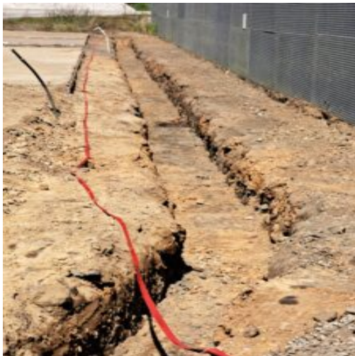
Trench has been excavated at the depth of 2ft
