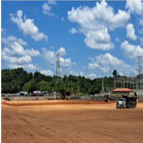
Placement of Lift at section 2 part 2
