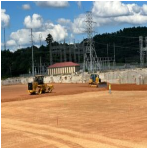
Placement of new lift in section 1
