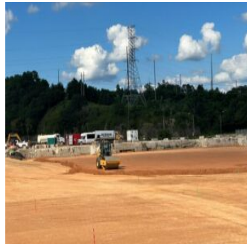
Placement of new lift in section 1 about to complete
