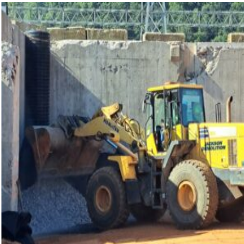
Placement of stone aggregate around the HDPE before the coverage of geo-fabric
