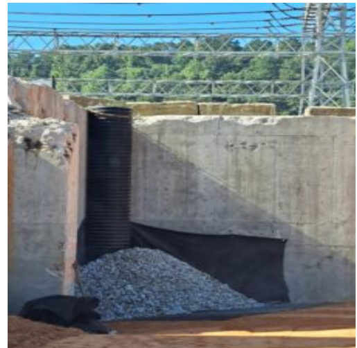
Placement of stone aggregate around the HDPE before the coverage of geo-fabric
