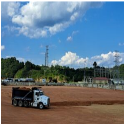
Placement of fill material in section 2 part 1
