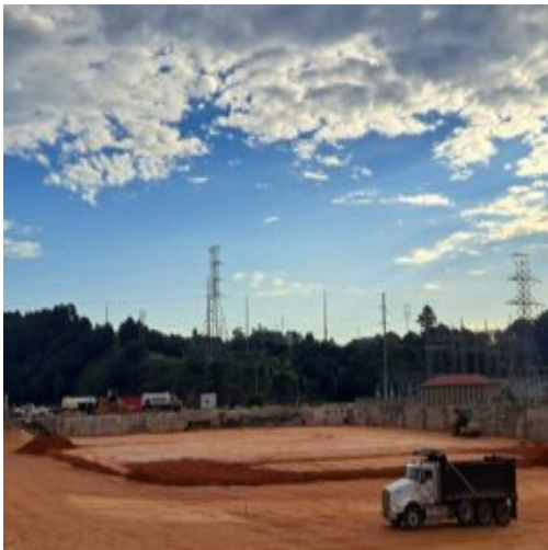
Started the placement of fill-material in section 2 part 1
