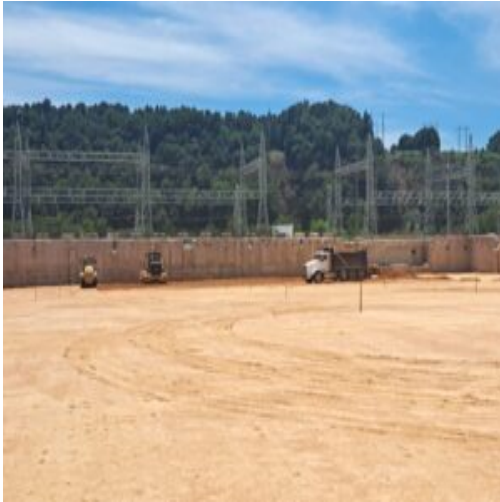
Placement of fill-material in section 2 part 1 basement area G7
