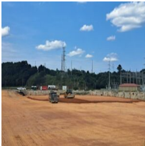
Placement of fill material in section 1
