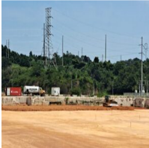
Placement of fill material in section 1
