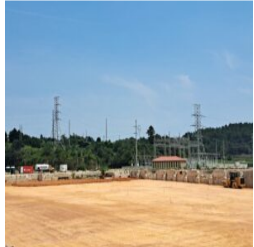
Started the placement of fill material in section 1
