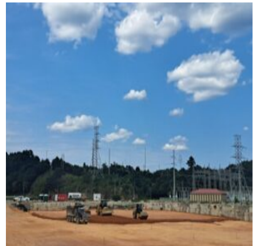
Placement of fill material in section 1
