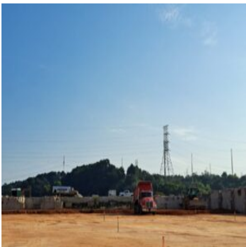
Placement of fill materials in section 1
