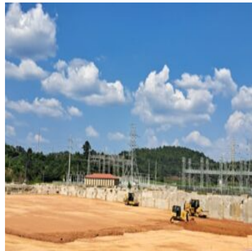
Placement of fill material in section 2 part 1
