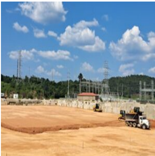
Placement of fill material in section 2 part 1
