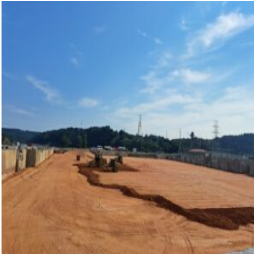
Fill-materials are placed in section 2 basement area G7 part 2
