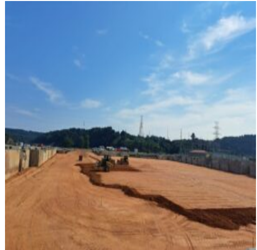
Fill-materials are placed in section 2 basement area G7 part 2
