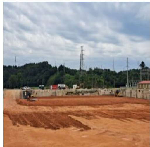
Placement of fill material in section 1 basement area B7
